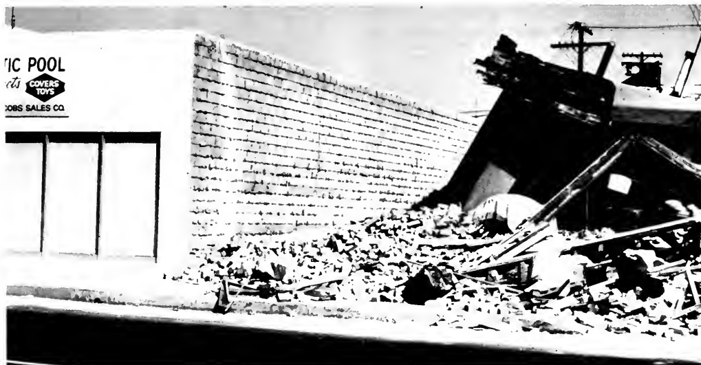
Photo 8. Contrast in response of masonry to seismic shaking. First Street in downtown San Fernando about 3 km south of Sylmar fault zone. A child was killed in the alder structure.
